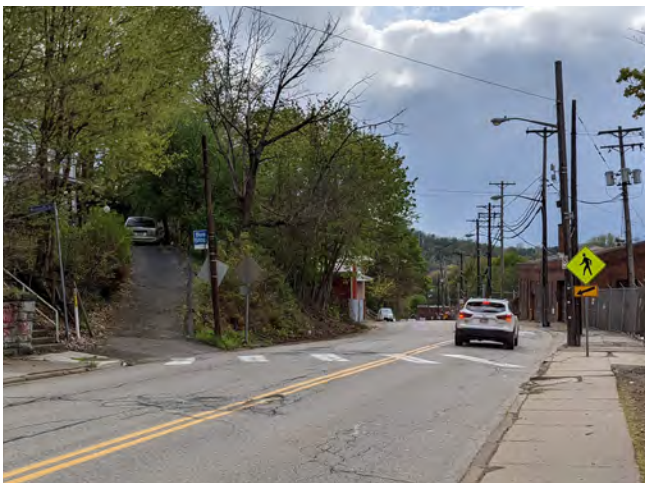
At the base of the Montooth Street Steps is the only marked crosswalk across Warrington Avenue leading to the station area. This non-signalized midblock crossing presents a safety concern for pedestrians accessing the station from Beltzhoover.
