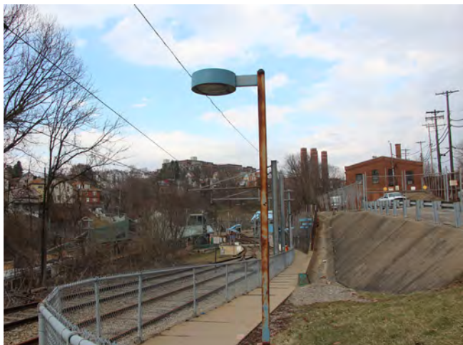
Along former Overbrook Line alignment (current staging track), the existing path leads down into the valley towards the light rail platforms. Stormwater is channelized behind the retaining wall and spills out onto the pathway.
