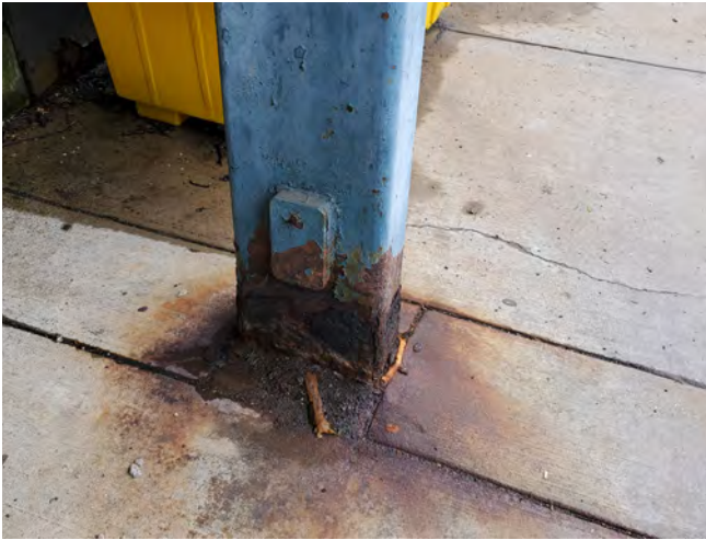
South Hills Junction Station is starting to show its age with rust and corrosion taking place in certain locations, especially where metal supports are embedded in walking surfaces that are routinely salted.
