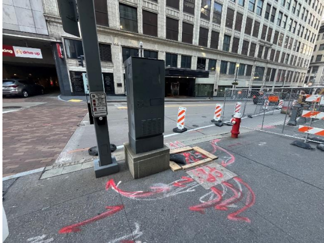
Image depicting a traffic signal box with pavement Markings placed in preparation for upcoming Work.
