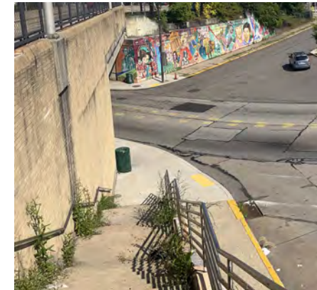
Fig. 28 View North Down the Sawyer Way Stairs
