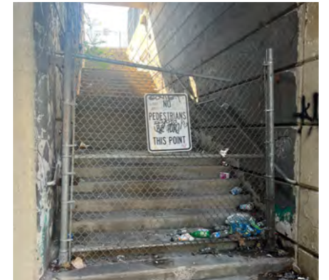
Fig. 30 View of Closed Staircase at Penn Avenue Under The Busway
