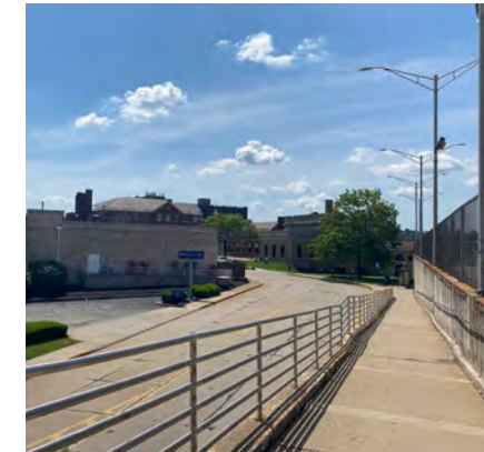
Fig. 29 View South Along the Sawyer Way Ramp
