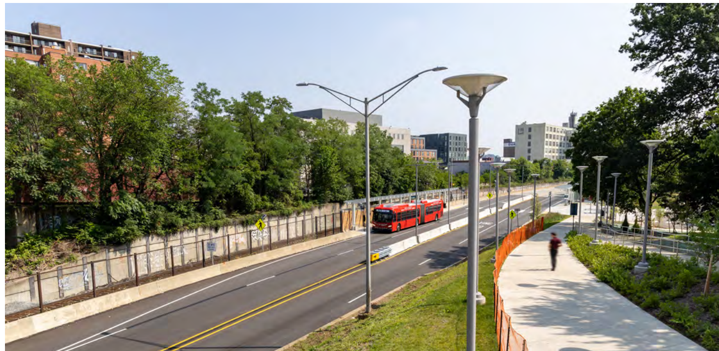
Fig. 7 Negley Station on the East Busway was reconfigured as recommended by the Negley Station Area Plan
