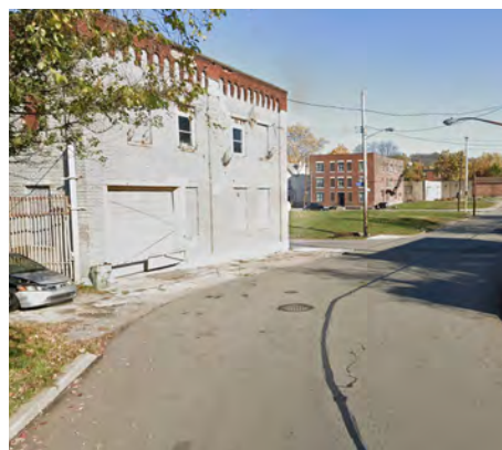
Fig. 31 View North Along Brushton Avenue Near the Park And Ride
