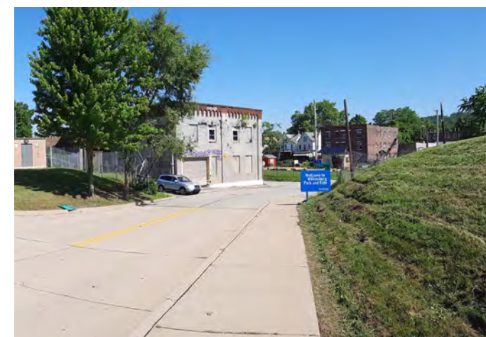
Fig. 34 View toward the Brushton Layover and the Brushton Avenue gateway
