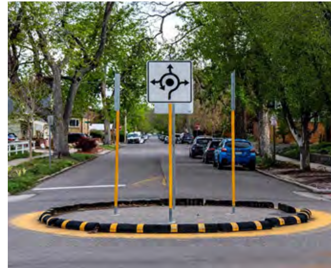
Fig. 21 Mini-Roundabout along Neighborhood Bikeway, Denver
