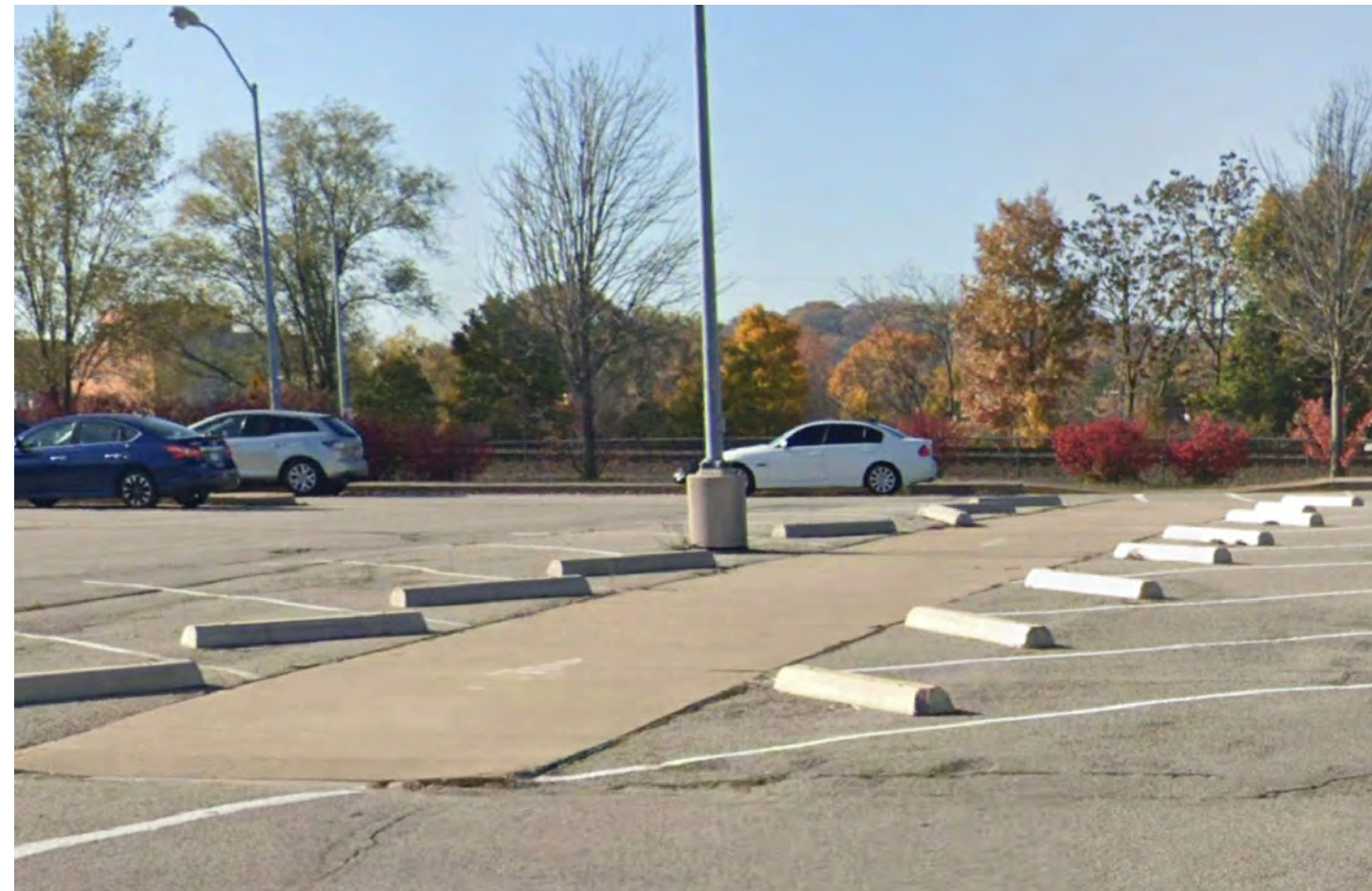
Fig. 17 Mid-Parking Lot Aisle to Rosedale Street and Hill Avenue Intersection
